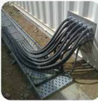
Cable Laying at Site
