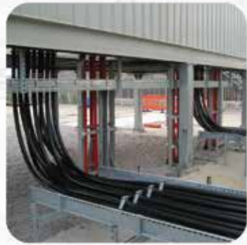
Cable Laying at Site
